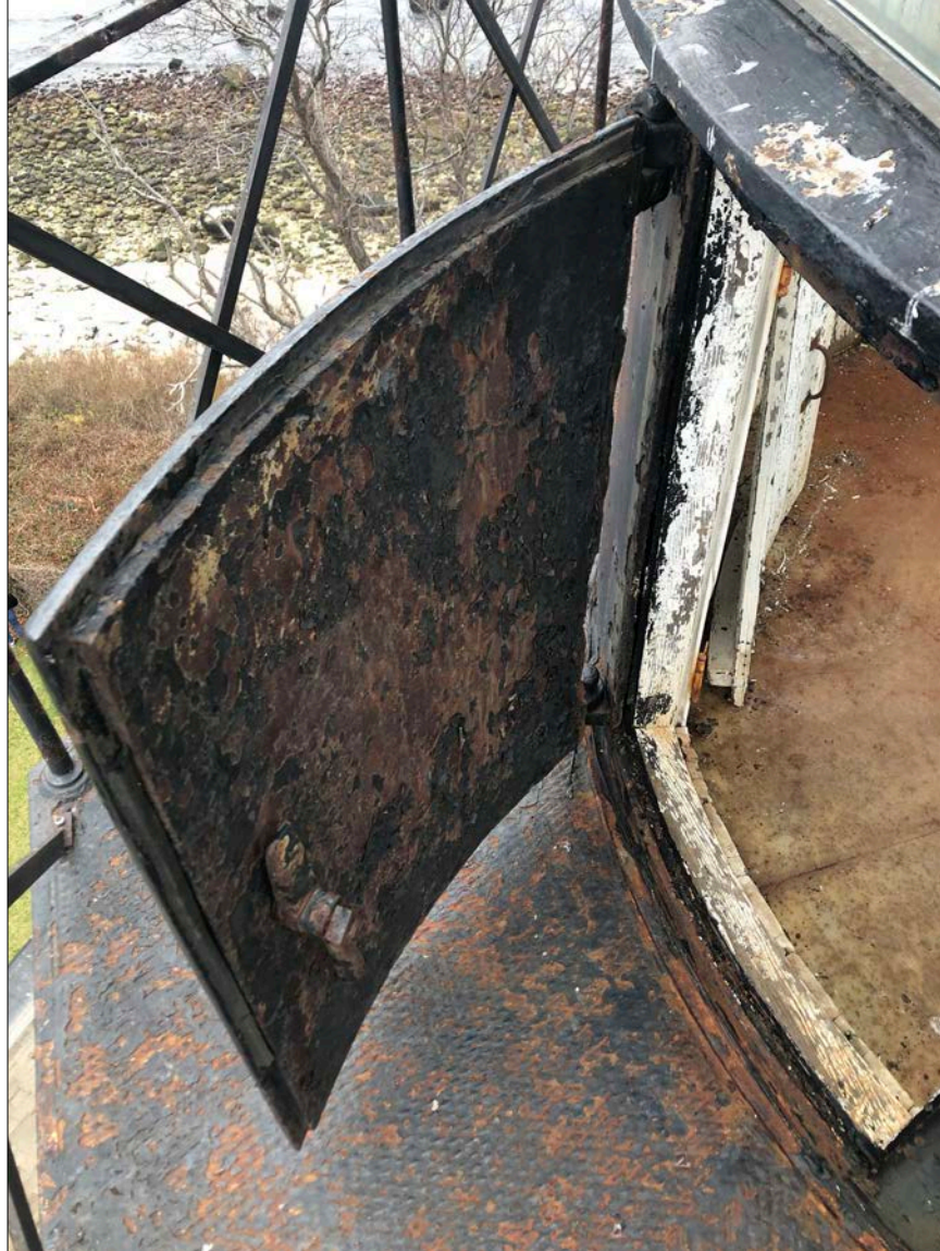
Photo 12. View of opened Lantern hatch, showing operation & hardware.
