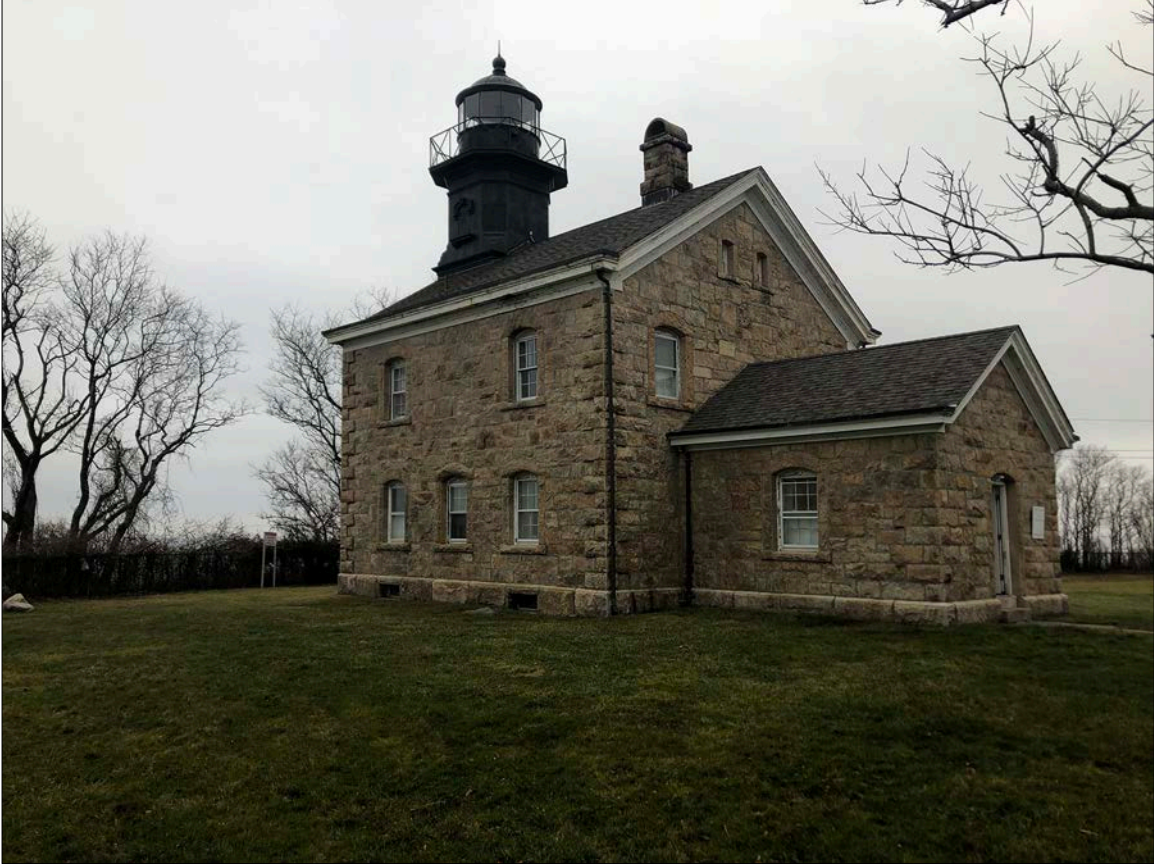
Photo 29. Quintessential view of Old Field Point Lighthouse, looking northeast. The building envelope, constructed principally of granite ashlar blocks, cast iron and simple gable roof forms is sound, though issues persist relating to stormwater management and – on the interior – structural framing.
