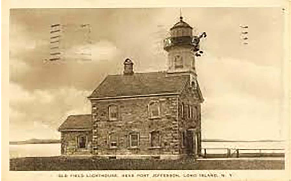
Image 1. Old Field Point Lighthouse, looking WSW, c.1868.
