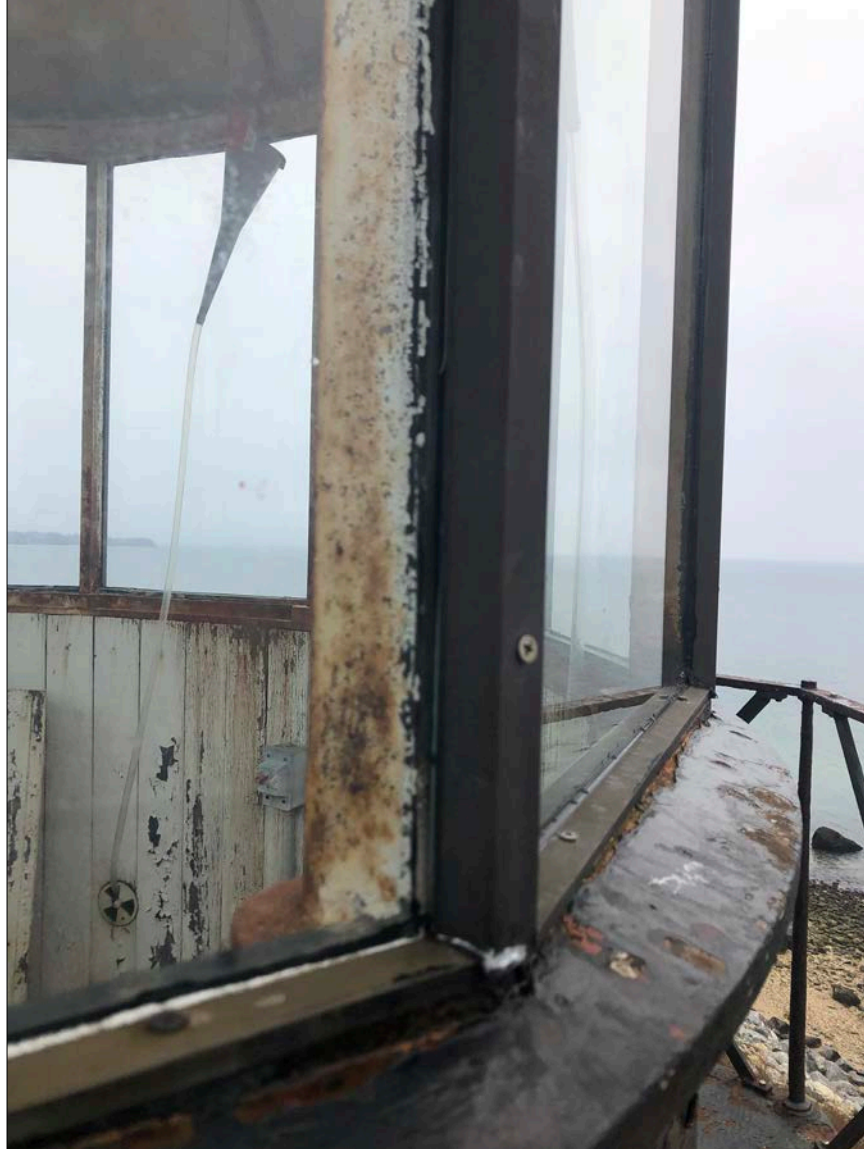
Photo 16. General view through exterior lantern glazing, looking northwest.
