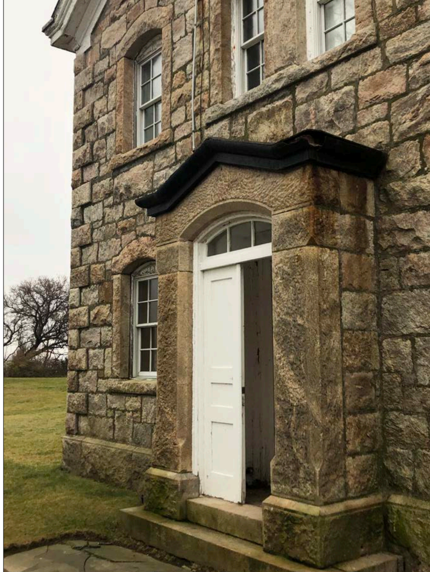
Photo 33. North facade and projecting Tower entrance, looking southeast.
